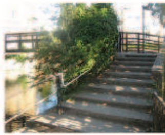
Steps - a barrier to movement
